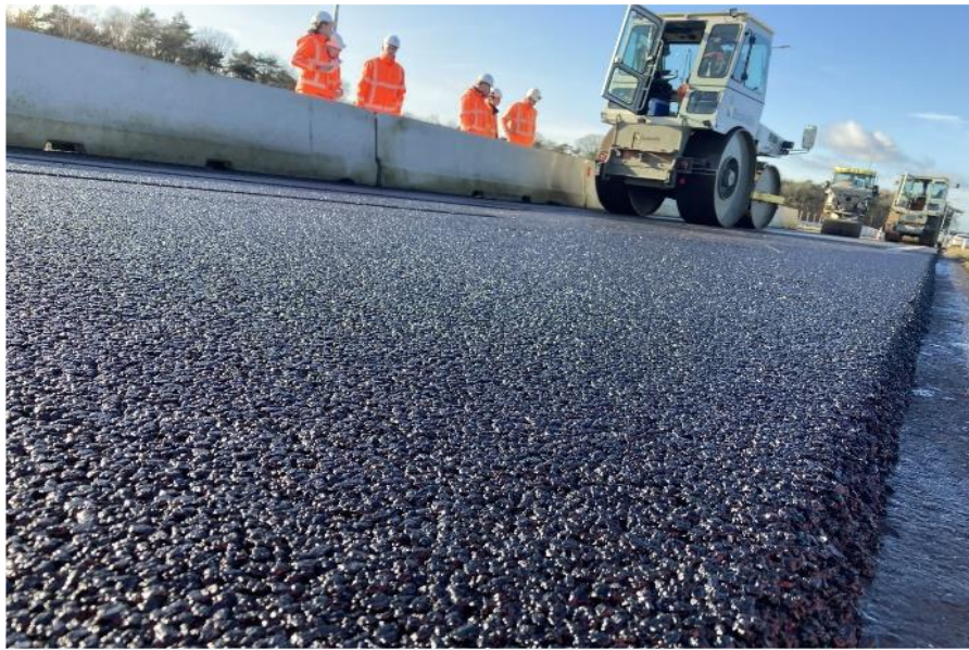
Fig. 2. Paving Circuroad test section A58 (December 2024).
