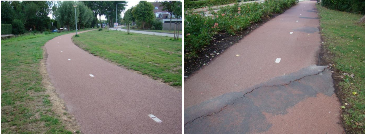
Figure 9 and 10: Bicycle path with polymer modified clear binder constructed in 2005. Apart from root and edge damage, no further damage in 2023.
