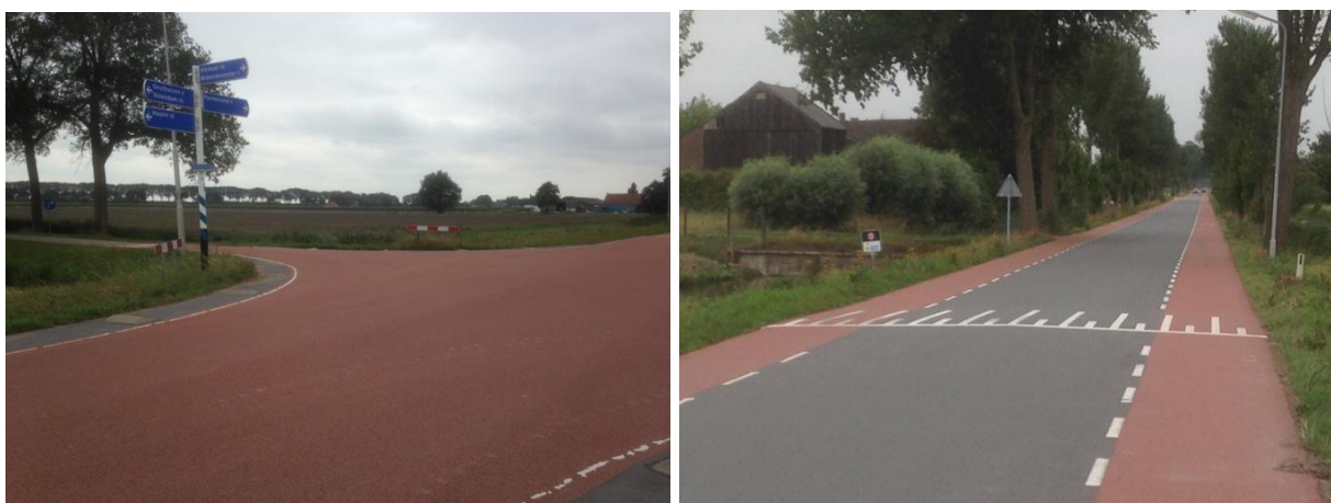
Figure 7 and 8: Red asphalt with polymer modified clear binder. Apart from edge damage, no further damage in 2019.
