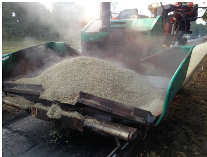
Figure 4: Applying white coloured asphalt.
