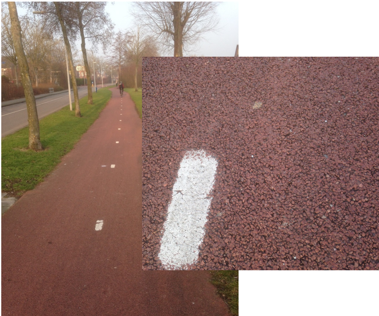
Figure 6: Impression bicycle lane after 11 years in service.
