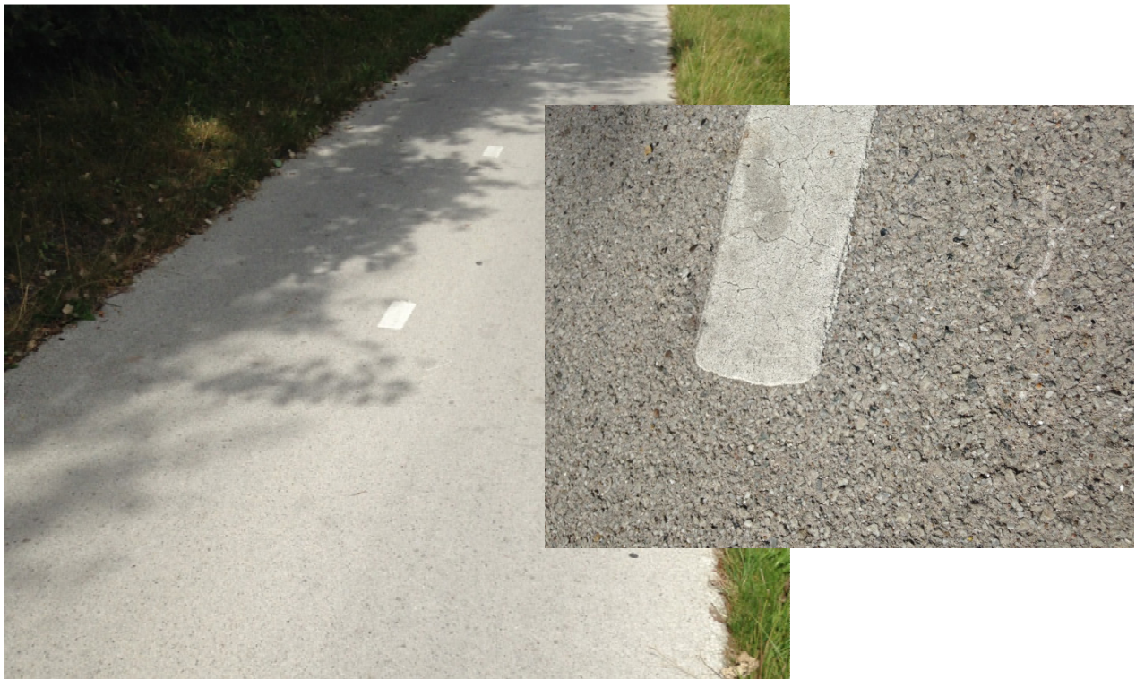
Figure 5: White coloured bicycle path after 3 years in service.
